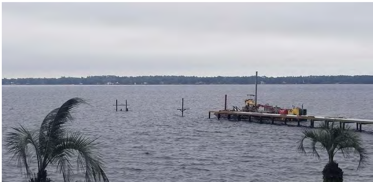
The dock repair progress
