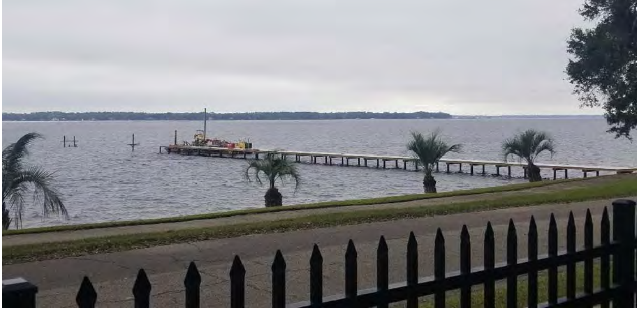
Pier repair progress
